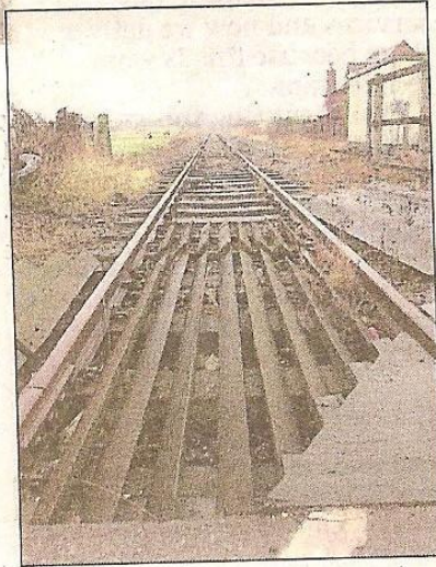
The disused line between Lichfield and Walsall could be up and running again by 2029 if regional transport chiefs' ambitions are realised. (AW776-1938LM)
